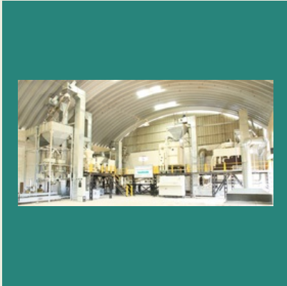
Seed Processing Plant
